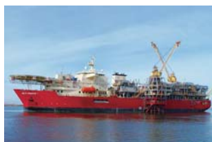
Floating production unit on the Phoenix Oil Field in U.S. Gulf of Mexico
