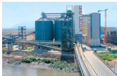
Flour mill, silos and port facilities of Interflour Vietnam Ltd.
