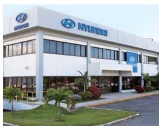
Headquarters of Hyundai de Puerto Rico
