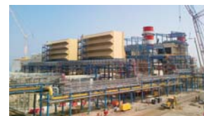
Construction is proceeding rapidly at Barka 3, with completion targeted in April 2013.
