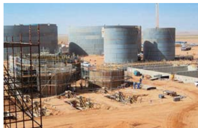
IPP project in Saudi Arabia (plant under construction)
