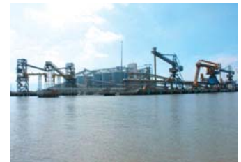
Port facilities of Interflour Vietnam Ltd.
