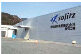
New processing plant of SOFCO Seafoods Inc.
