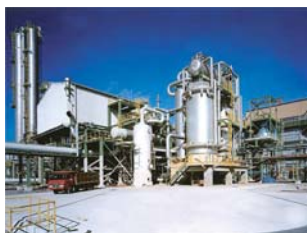
Methanol manufacturing facilities in Indonesia
