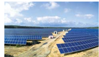
24MW solar power plant in Germany
